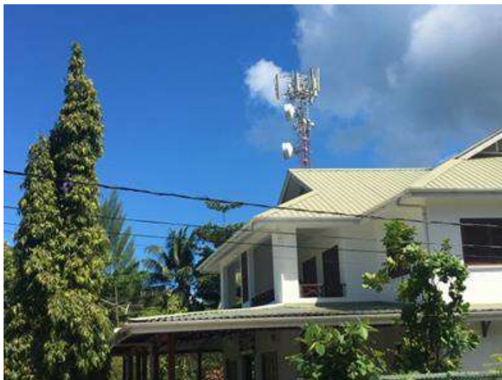
Figure 112 – Grand Anse: base station (Airtel) adjacent to MP4 location
