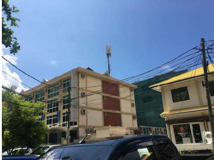
Figure 91 – Sunshine House: identification of base station at MP1
