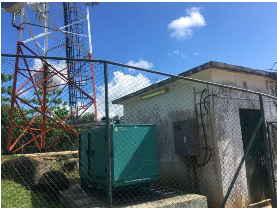
Figure 7 – North East Point: At MP1 location
