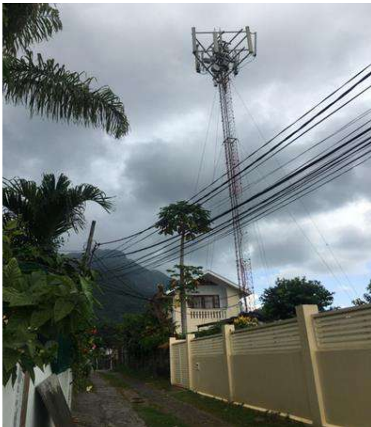
Figure 77 – Plaisance: at MP2 location
