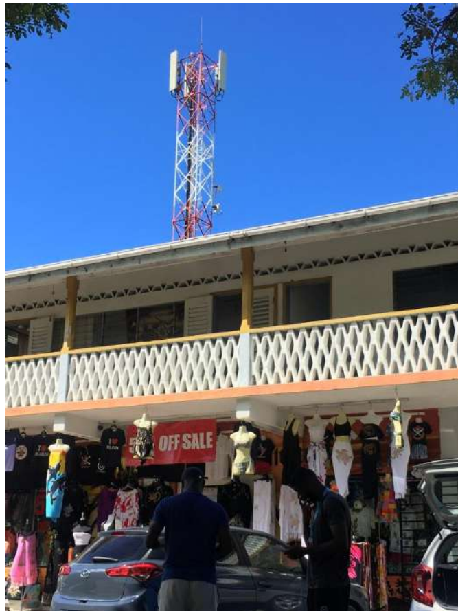
Figure 109 – Grand Anse: MP2 location (CWS)
