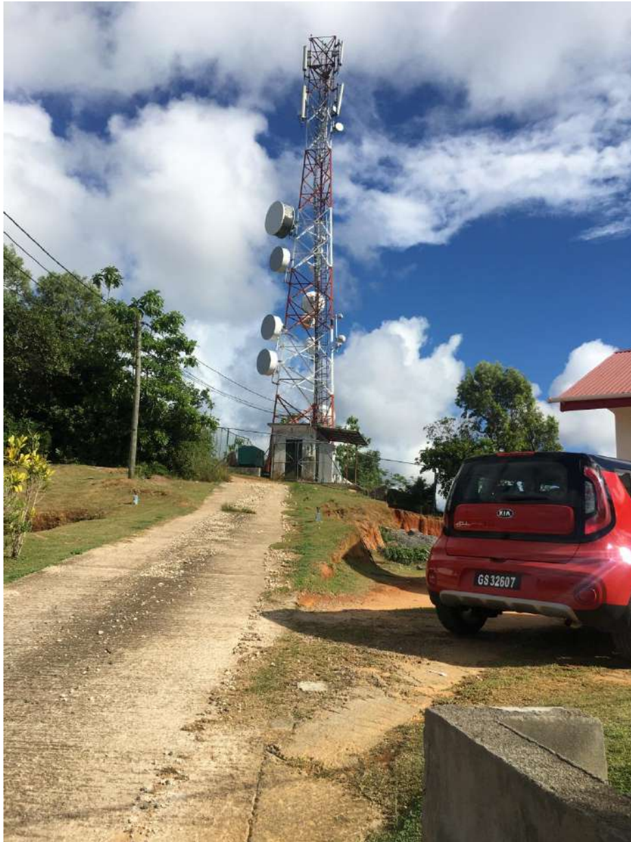
Figure 8 – North East Point: At MP2 location
