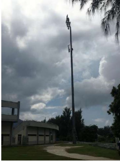
Figure 85 – Roche Caiman (RC1): MP1 location
