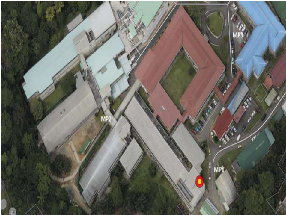
Figure 65 - Seychelles main hospital: measurement points (WebGIS)
