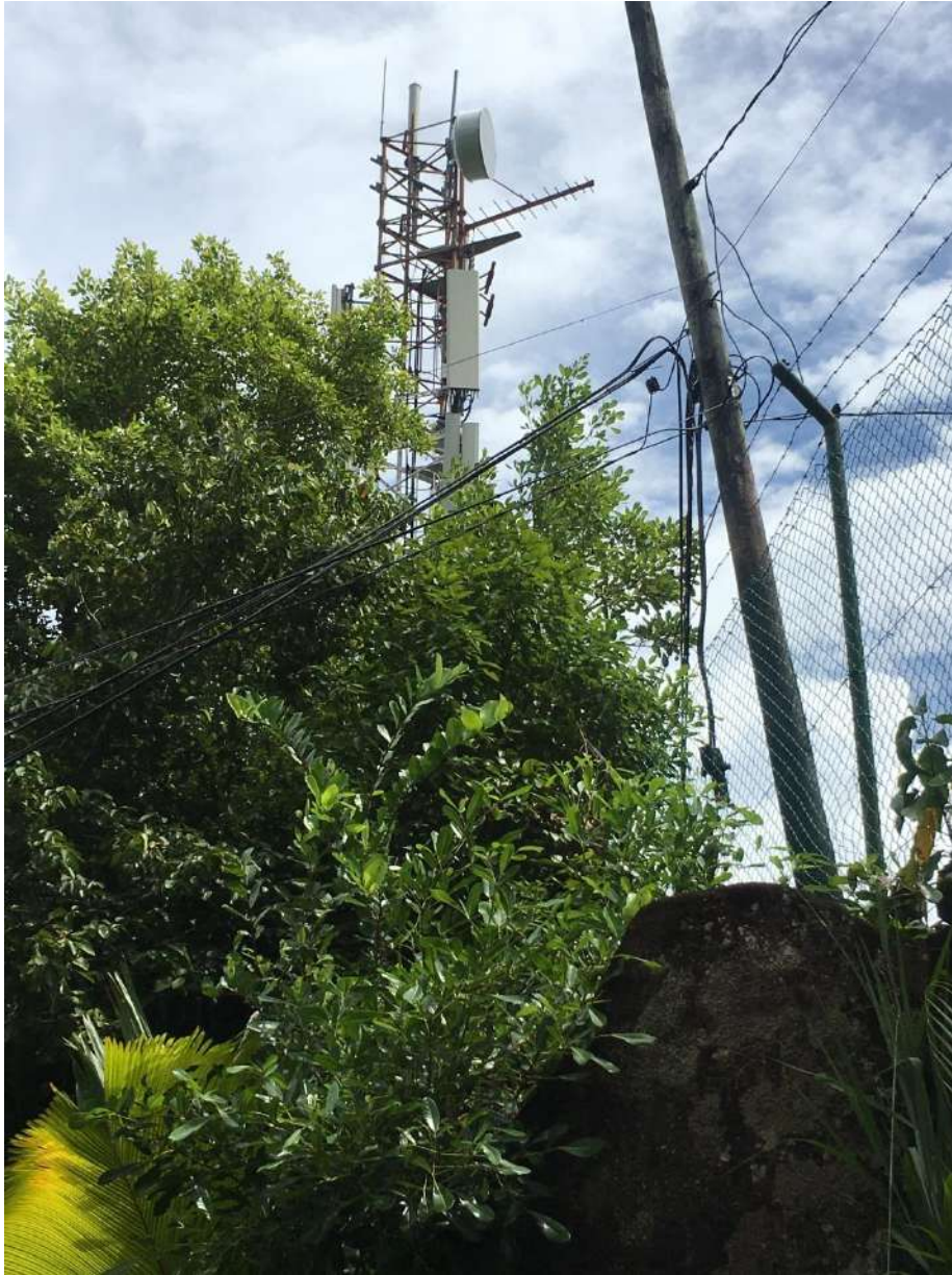
Figure 16 - Bel Ombre (DZ): MP2 location
