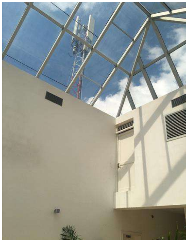
Figure 92 – Sunshine House: identification of base station at MP2
