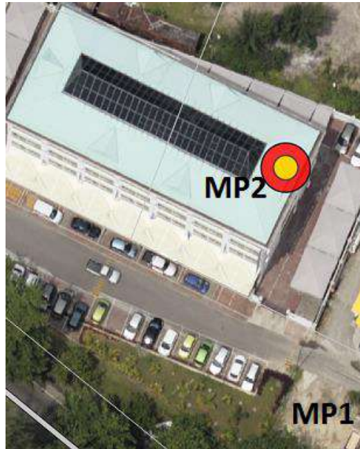
Figure 89 – Sunshine House: measurement points (WebGIS)
